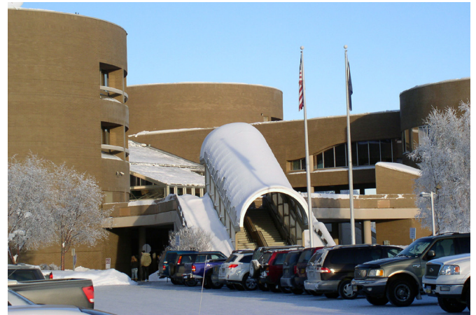
Stair to Main Entry, Level 2
